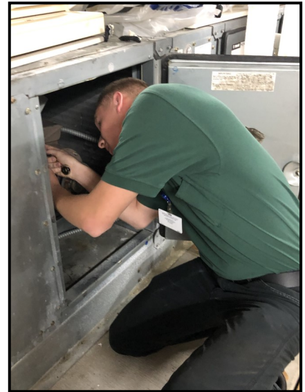
Aden Leisey, EL, Plumbing, Moravian Manor
