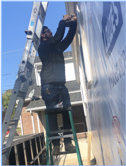
Mike Weaber, PA, Carpentry, Allen Restorations
